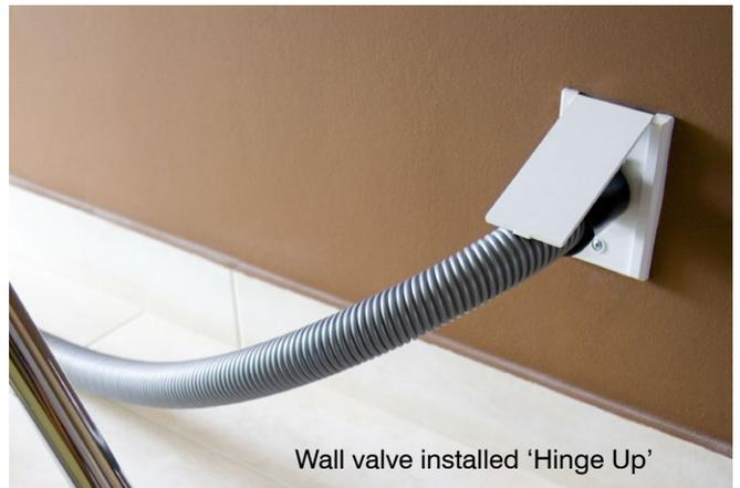
Simply screw the wall valve to the mounting plate to complete the task. If the PVC ducting is directly behind the screw locations be sure to use short screws that will not reach and puncture the duct.
